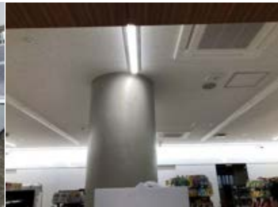
30-40 kw for usage such as Air Conditioning
