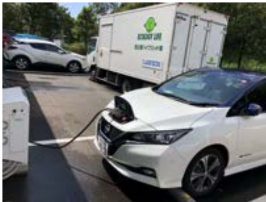
5.6 kw for storage
